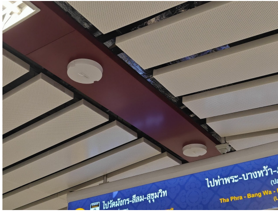
Fig. 3: DAS nodes deployed in pairs for up to 4T4R operation application records the reported modem parameters every 0.5-second intervals. The log file is then opened in the AirScreen software, where relevant parameters such as the Reference Signal Received Power (RSRP), Signal to Interference Noise Ratio (SINR), and Modulation and Coding Scheme (MCS) are selected and exported with corresponding timestamps to a CSV file. The CSV file is then opened in Microsoft Excel for data analysis and figure construction.
