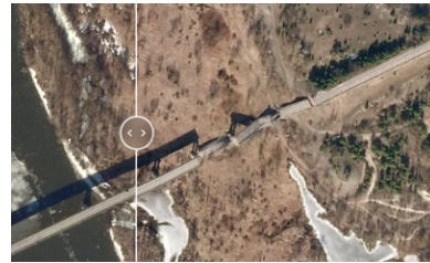
(b) Destroyed road at Kamaryn-Slavutych.
