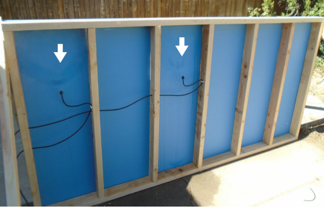
Fig. 4. Photograph of partially completed test structure used to evaluate acoustic detection of water leaks behind gypsum board. Arrows show the fixed locations of two independently activated simulated leaks. A second gypsum board (not shown) seals the structure for testing.
