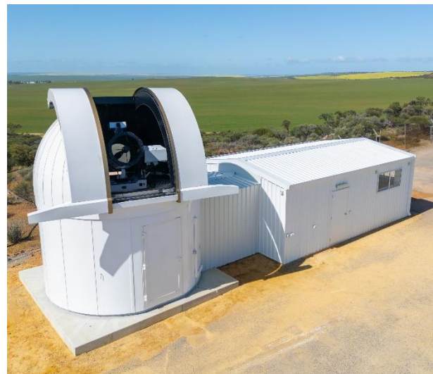
Fig. 6. Photo of TN-2 facility at the Yarragadee Geodetic Observatory.
