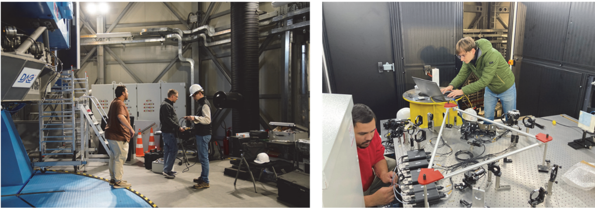
Figure 6. The PLACID team from the University of Bern started the on-site cabling and interfacing work during the early July 2025 campaign.
