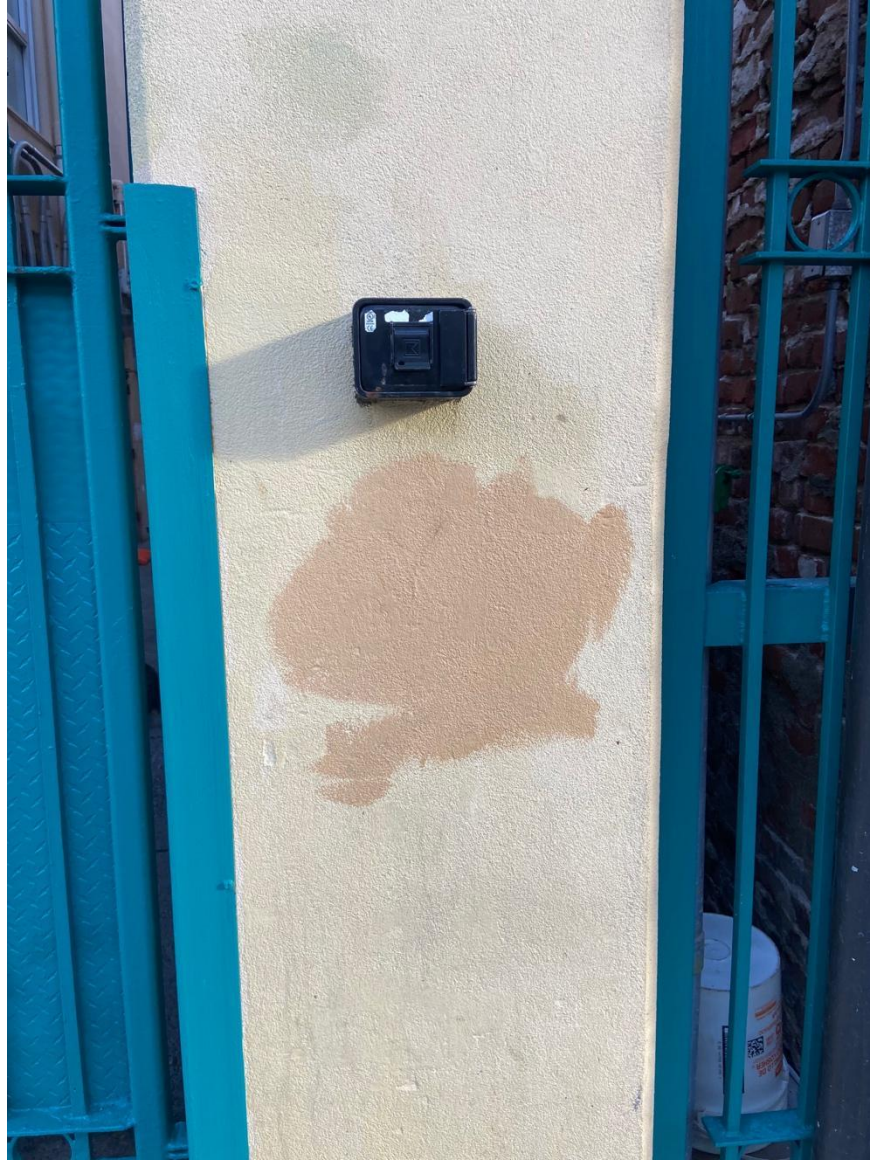
Figure 7. Wall with covered paints.
